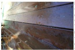
Boards that have propensity to cup usually do so for a variety of reasons, none of which have to do with the fastening systems. No fastening system can prevent, delay, or otherwise stop a board from cupping except over the joists - by virtue of the fact that the cupping occurs between the joists.
